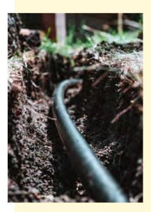
**Note on supply lines:** You have a few options for running supply lines from your water source to your gardens. In many cases, blank irrigation tubing and/or garden hoses are used, though some setups use PVC pipe. If you're unable to permanently connect to your water source, using a garden hose as your supply line allows you to easily connect and disconnect the system.
