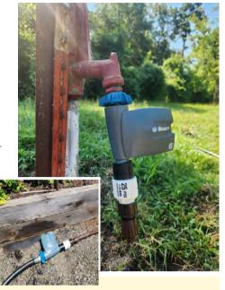
**Tip:** Be sure that the timer is located closer to the spigot with the pressure regulator coming after it. This reduces the strain on the pressure regulator.
